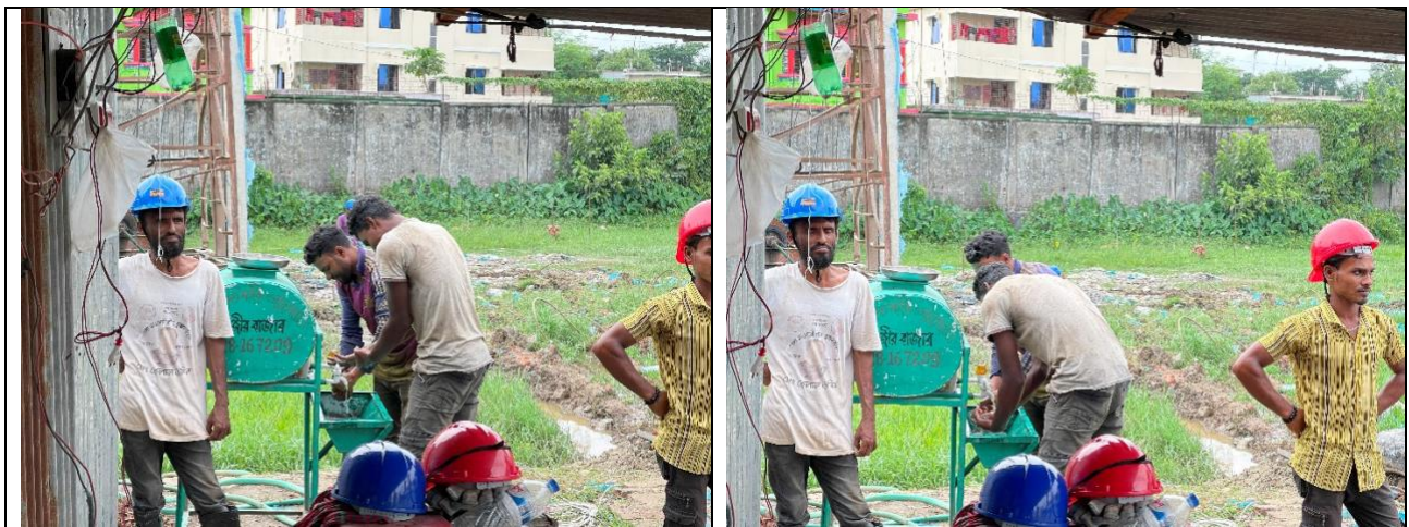
Hand Wash Facility at Medical Center Construction, Akhaura Land Port
