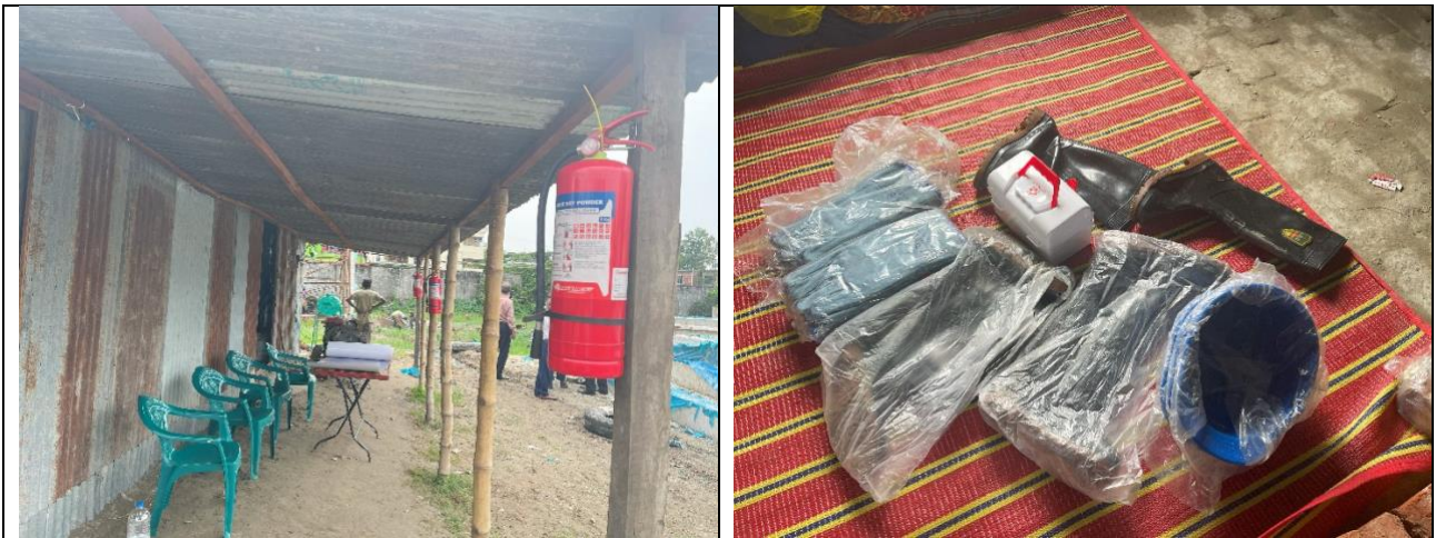
PPE and Fire Extinguisher at Medical Center Construction, Akhaura Land Port
