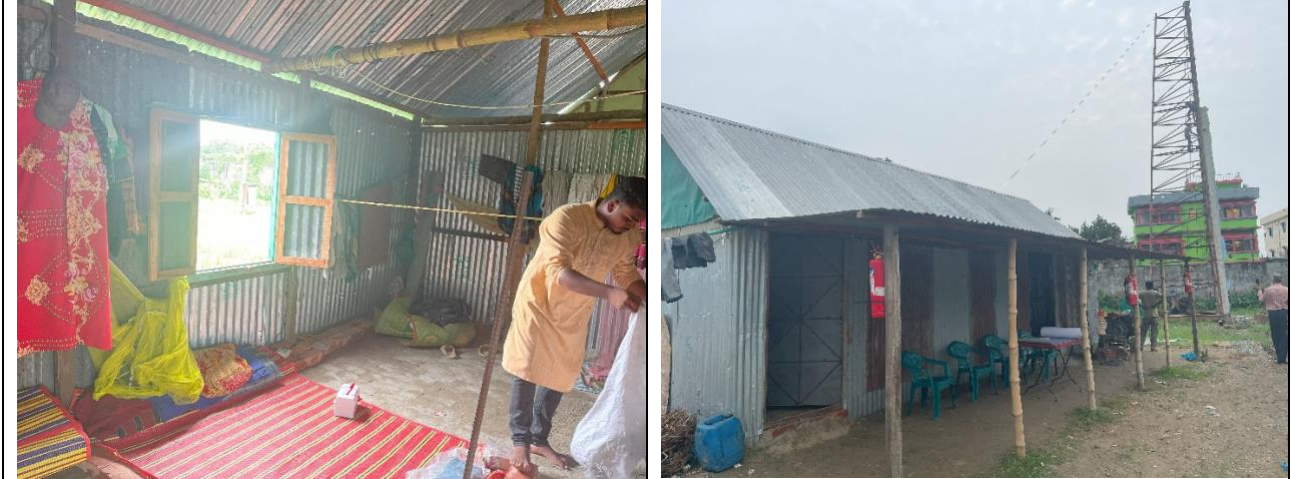
Workers Living Facility at Medical Center Construction, Akhaura Land Port
